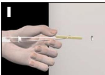
Drill appropriate size hole. Hold metal channel flat alongside plastic straps & slide channel through the hole.
